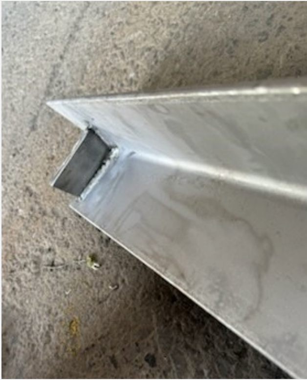
Flat bar can also we welded to the bottom end of the lintel to form a “kick out or stop end” to divert the water.
