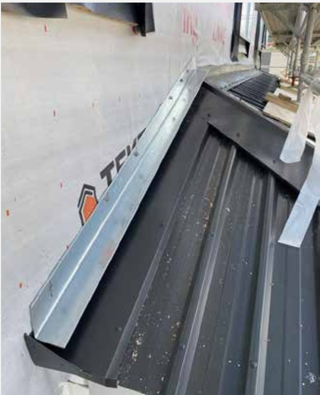
Flat bar can also we welded to the bottom end of the lintel to form a “kick out or stop end” to divert the water.
