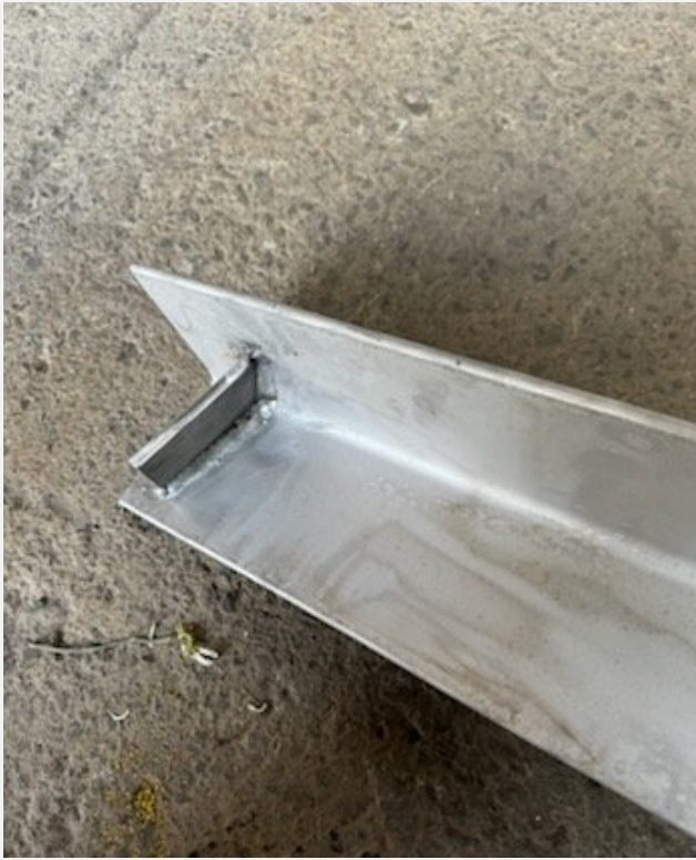
Flat bar can also we welded to the bottom end of the lintel to form a “kick out or stop end” to divert the water.
