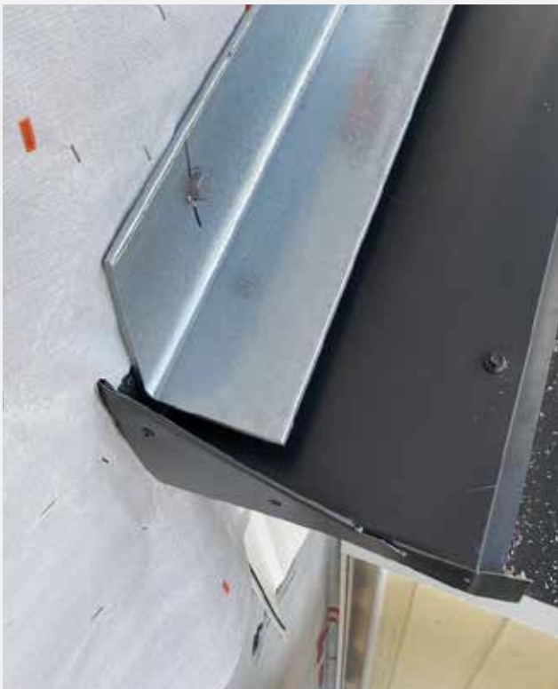
Flat bar can also we welded to the bottom end of the lintel to form a “kick out or stop end” to divert the water.
